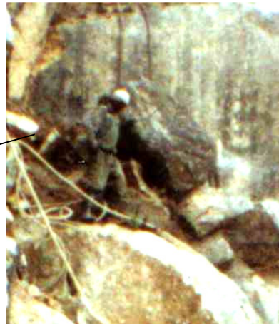
Figure 2: Construction on an active roadway, which is sometimes necessary when there is absolutely no alternative access, increases the rockfall hazard many times over that for slopes without construction or for situations in which the road can be closed during construction.
